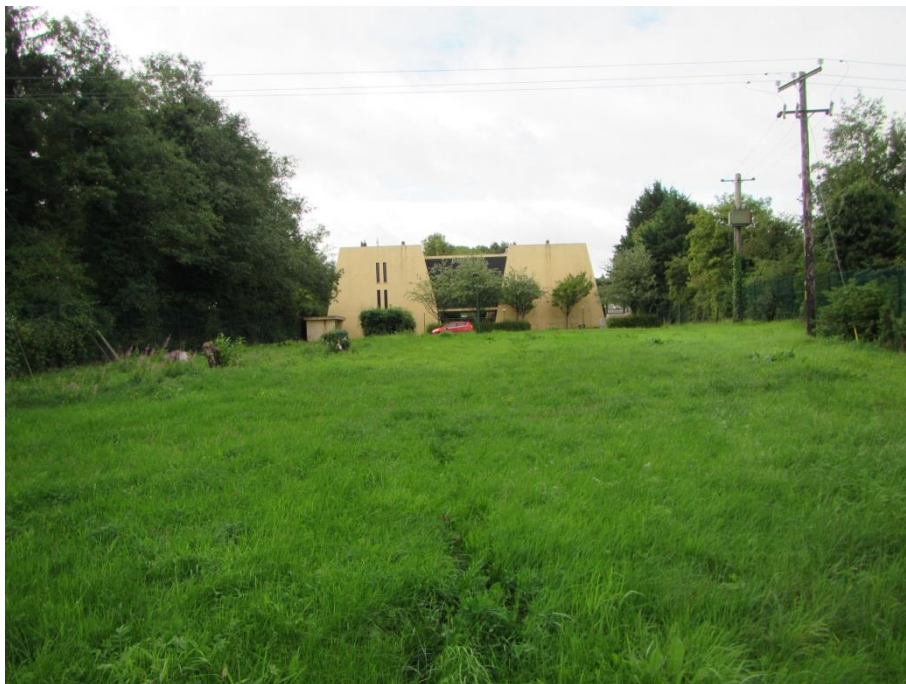
Figure 13-6 Looking south towards OPW building
