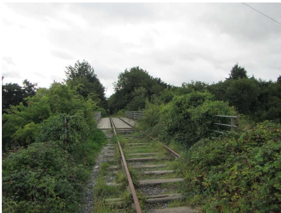
Figure 13-17 The protected structure railway bridge (NT025-173)
