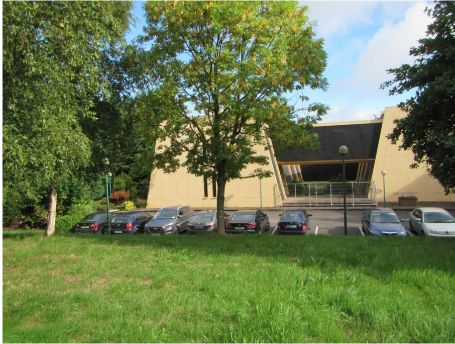
Figure 13-5 Looking north across OPW building
